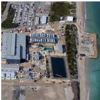
Perth Seawater Desalination Plant, Australia VLT® drives and softstarters were chosen to run pumps when The Water Corporation of Western Australia – one of Australia's largest and most successful water service providers – invested $387 million Australian dollars in Perth Seawater Desalination Plant – the largest of its type in the Southern Hemisphere. The company provides water and wastewater services to the burgeoning city of Perth and hundreds of towns and communities spread over 2.5 million square kilometres.
