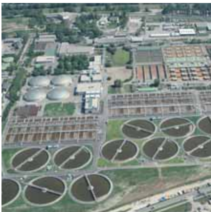
Vienna's Main Sewage Treatment Plant, Austria At Vienna's lowest point, where the Danube Canal meets the Danube, lies Vienna's Main Sewage Treatment Plant. Here around 90% of Vienna's wastewaters is purified. VLT® Drives were chosen to operate the pumps that handle more than 500,000 cubic metres pr. day, which corresponds to a flow of a medium-size river. It takes about five hours for the waste water to pass through the mechanical and biological purification stages before it is purified and discharged into the Danube Canal.
